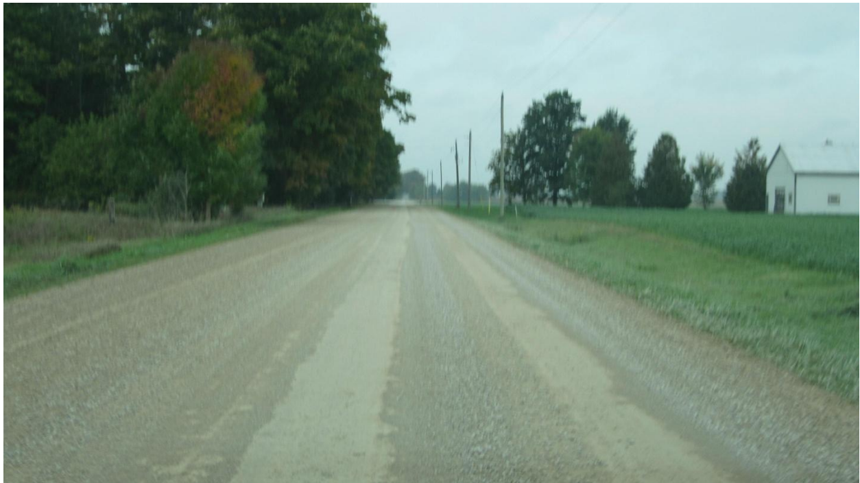
Figure 15: View of collision site looking west, taken the day after the collision. There are only two wheel-tracks visible on the road surface when, typically, there are three such tracks.
