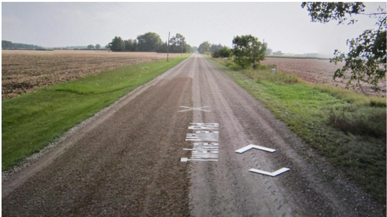
Figure 13: Google Maps view looking east from a short distance east of the area of impact. There is clear evidence that a fresh layer of gravel had been deposited in the westbound lane.
