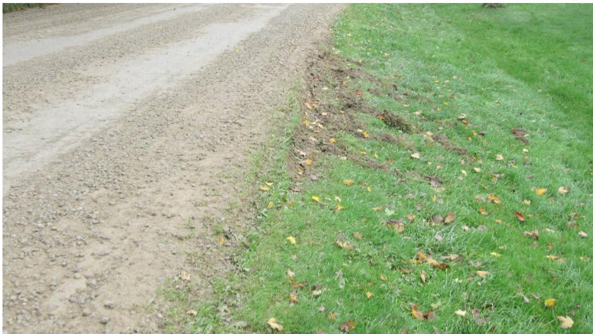
Figure 25: View, looking west, at the tire marks on the north roadside that were caused by the school bus just before in crossed to the south side of the road.
