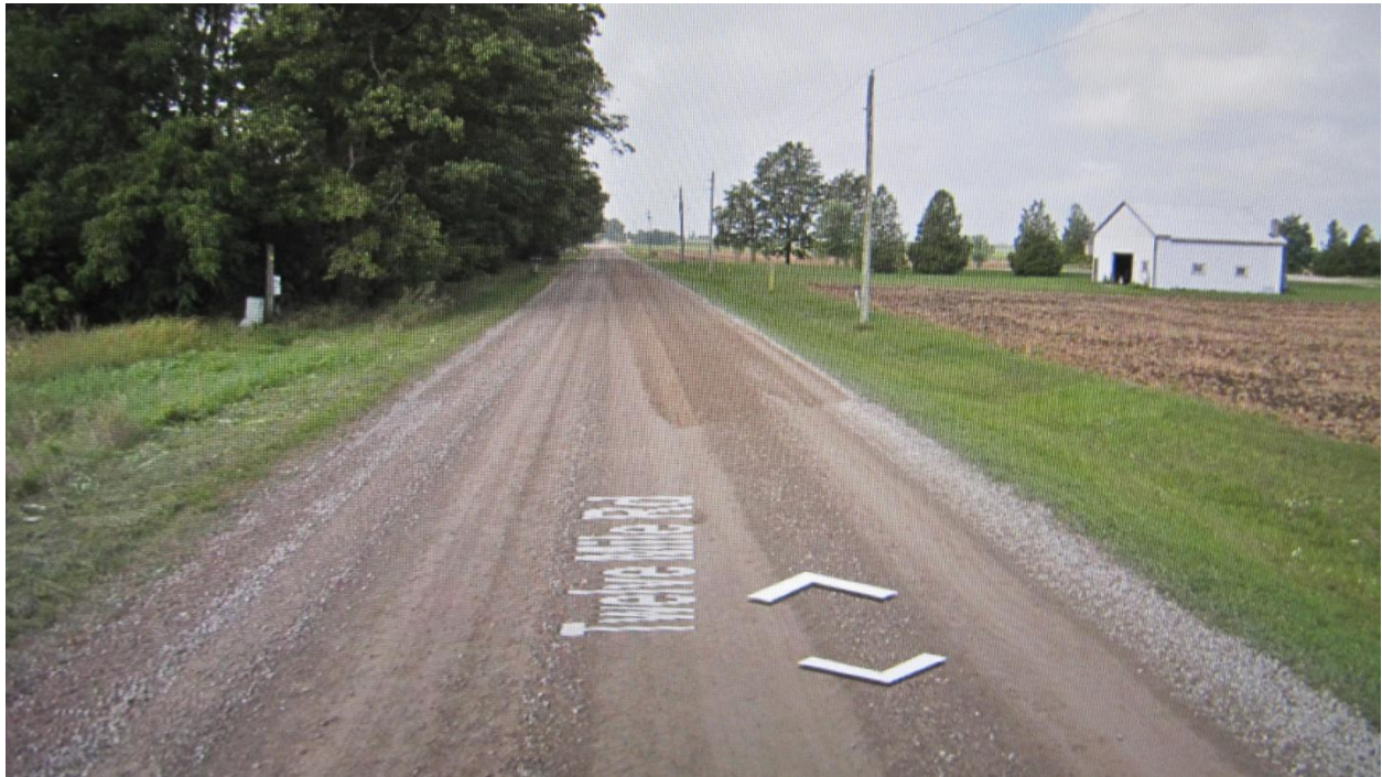
Figure 14: View looking west, showing the fresh layer of gravel that has been deposited for a short distance of the westbound lane.
